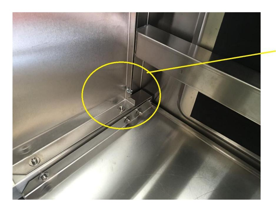
The hole for left panel and sink top is ready, continue to fix four holes, Hole 1, hole 2, hole 3 and hole 4.
